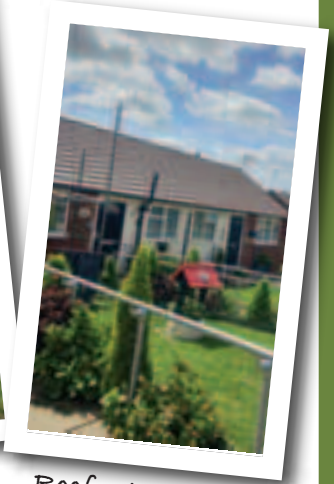
Roofs at Edward Court (After)
