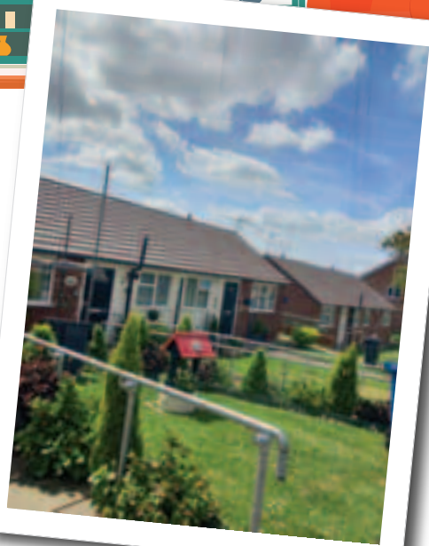
Roofs at Edward Court (After)
